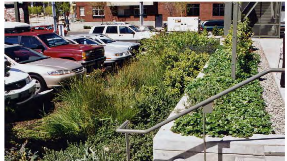
Fig 5 Blue-green roof and raingarden, Portland, Oregon
